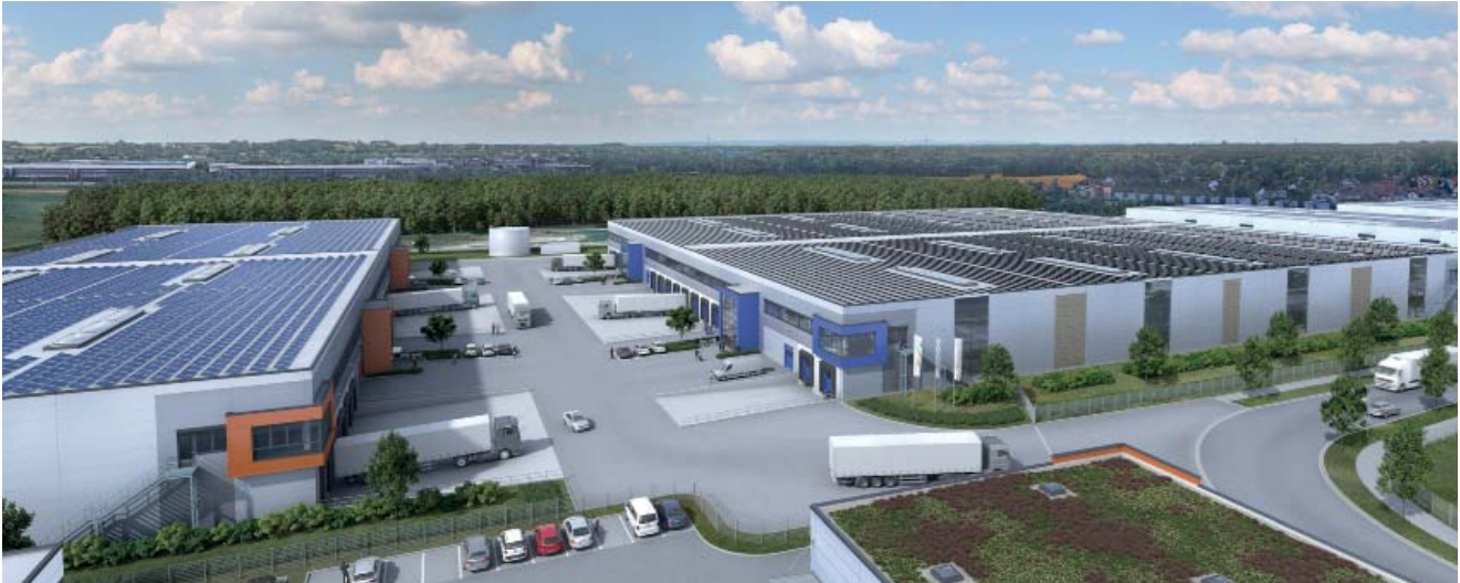
MayTec GmbH plant in Olching
